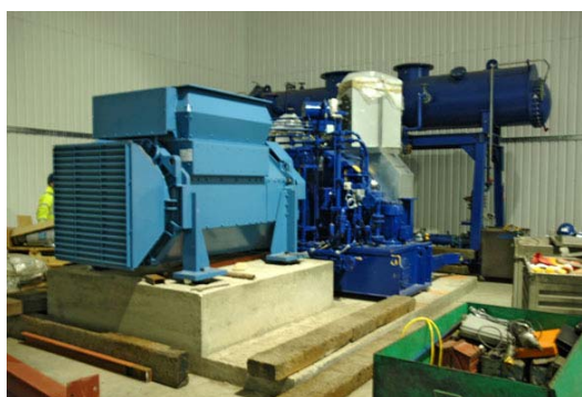
Figure 4. Construction of the turbine/generator and control systems for a comparable plant.
